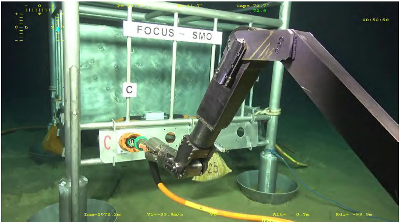
Figure 11: connection of the umbilical from the cable-end module, via the ODI wetmate connector to the Y-junction box using ROV Victor6000 (manipulator arm Maestro).
