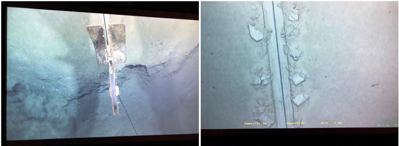
Figure 13: (left) blade of the plow in rough terrain (obstacle avoidance mode); (right) plow track in soft, flat sediments, after successful burial of the 9mm diameter fiber optic cable (note small fish at right).
